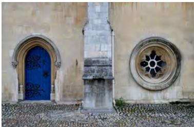
The Crypt Gallery entrance in Cathedral Close
